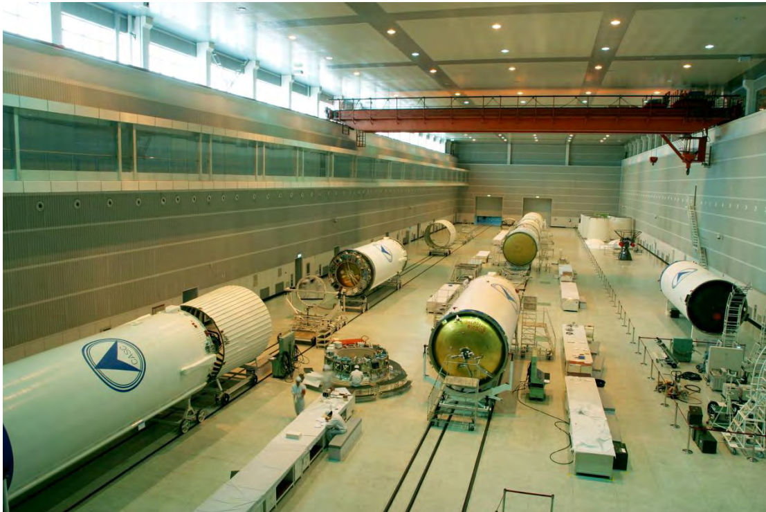
Figure 1-4 Long March LV Assembly and Test Workshop
